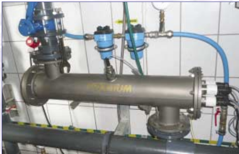
Typical Titanium AOP installations
