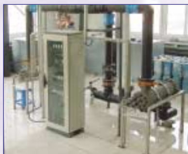
Typical Titanium AOP installations
