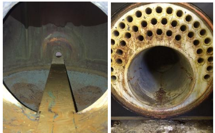
Internal images of the calorifiers prior to removal
